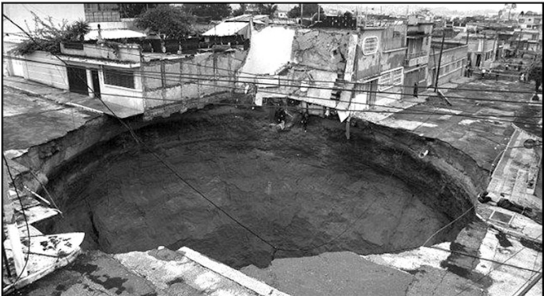
A massive sinkhole that swallowed a whole building recently.
