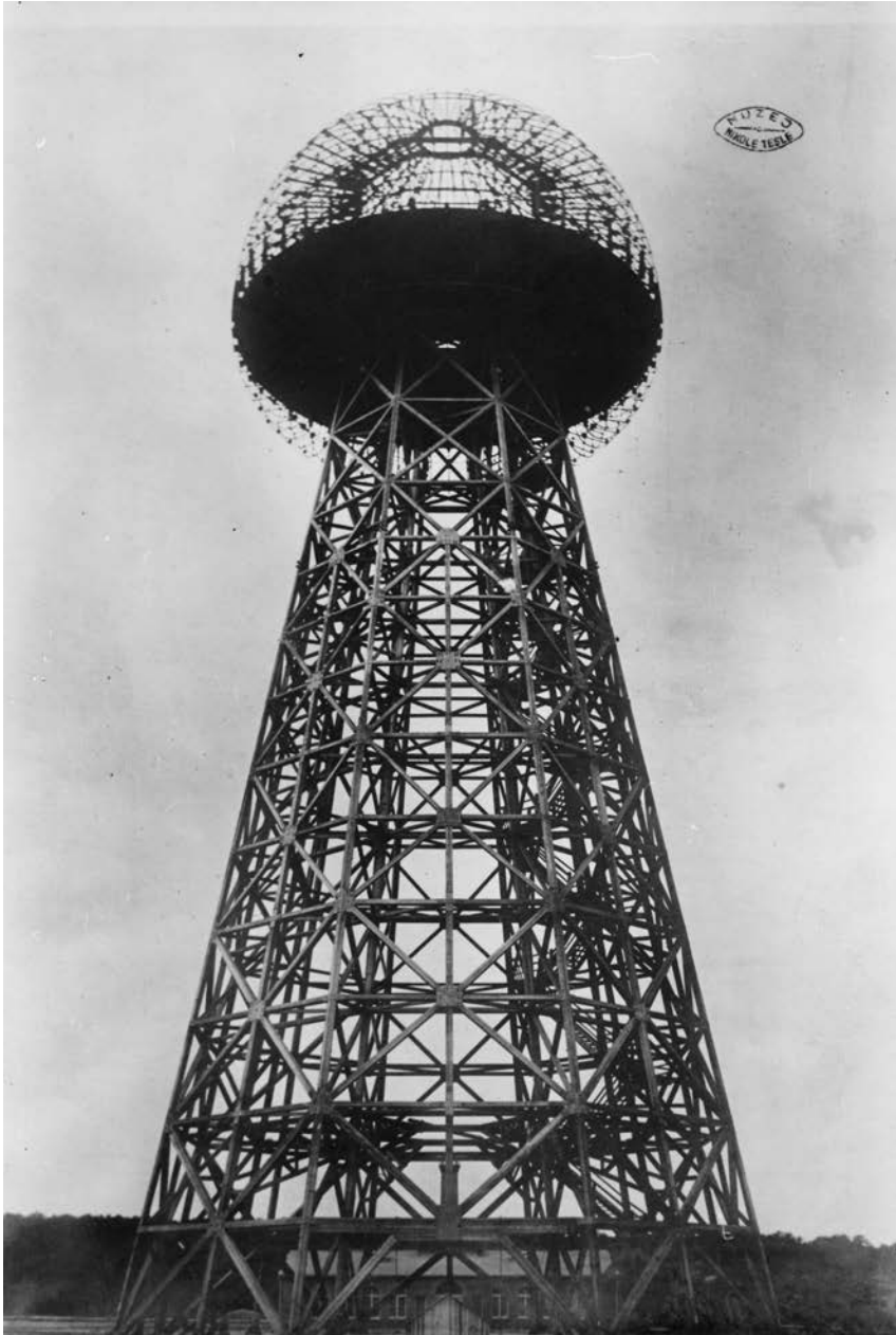
FIGURE 14.7. The tower at Wardencliffe showing hemispherical terminal on top. From KSP, Smithsonian Institution.
