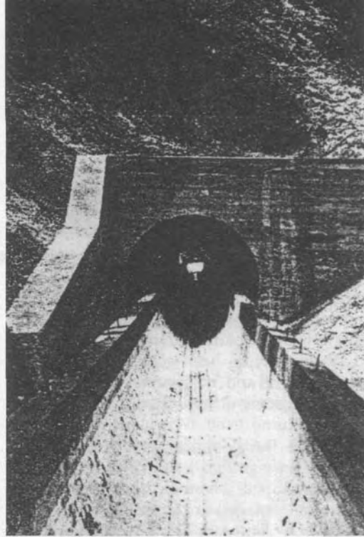
Fig. 12.3 Egg-shaped form of log flume
